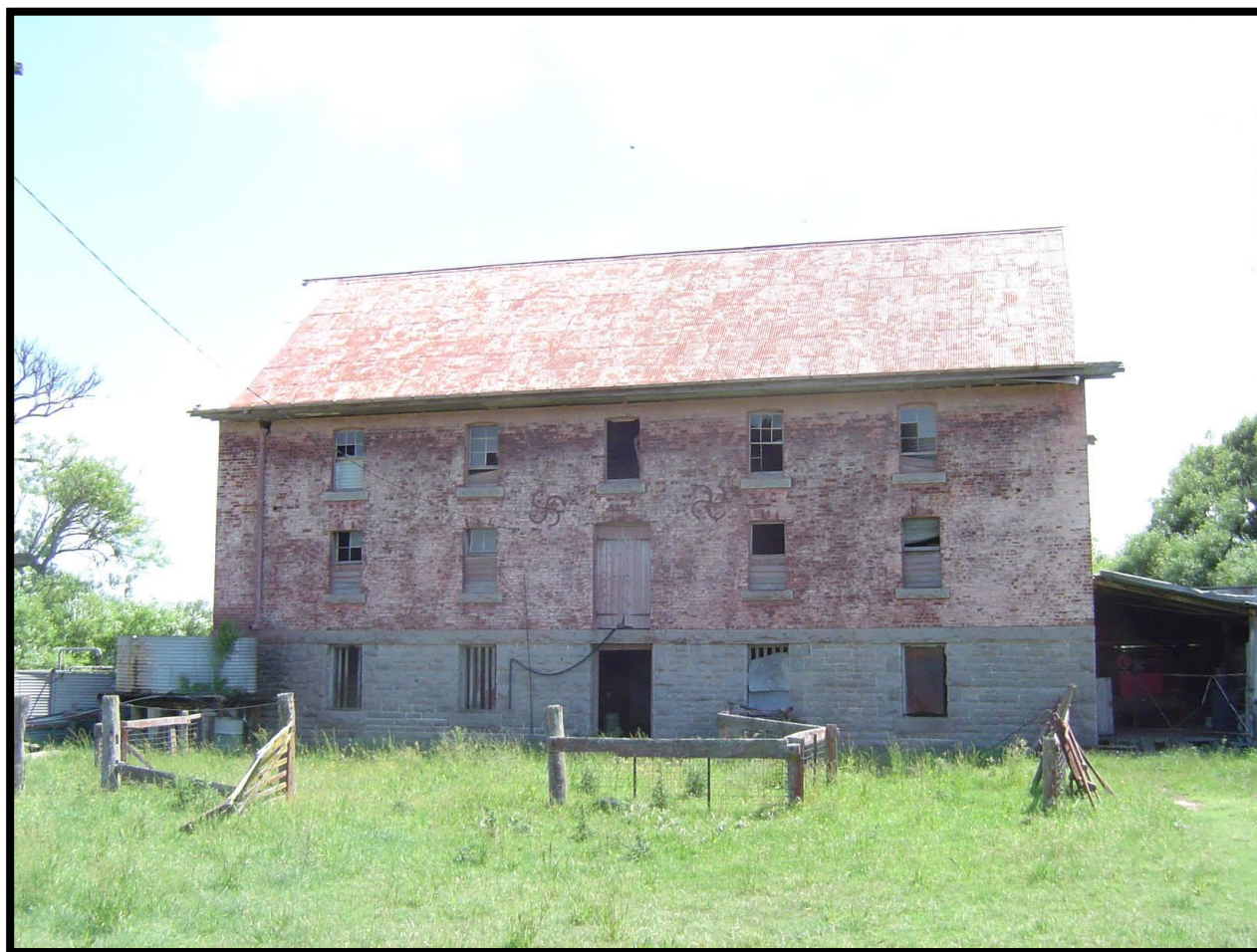
The Jembaicumbene Mill in 2008
