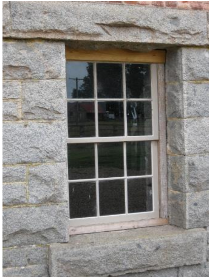
Ground floor window with reproduction sash window fitted 2012
