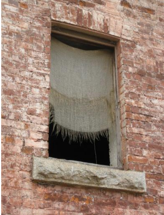
Upper floor window fenestration as found in 2008
